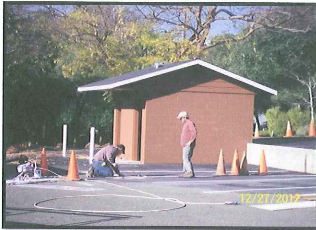
Progress continues on our new Marina bathrooms.
