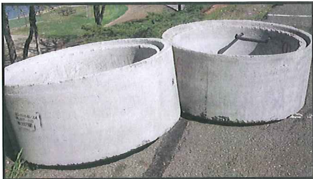
Each of these are 2' extensions, both manholes were raised 4' (Big Beach area).
