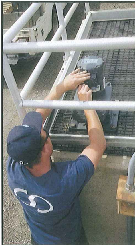
Alumn motor/mixer at Treatment Plant was rebuilt and installed .
