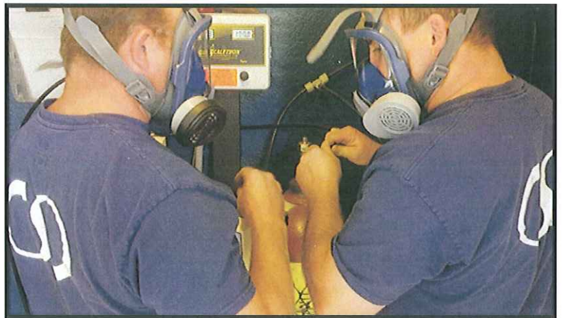
Annual maintenance performed at Well 4 on the CO2 that includes changing regulator lines and rotometer.
