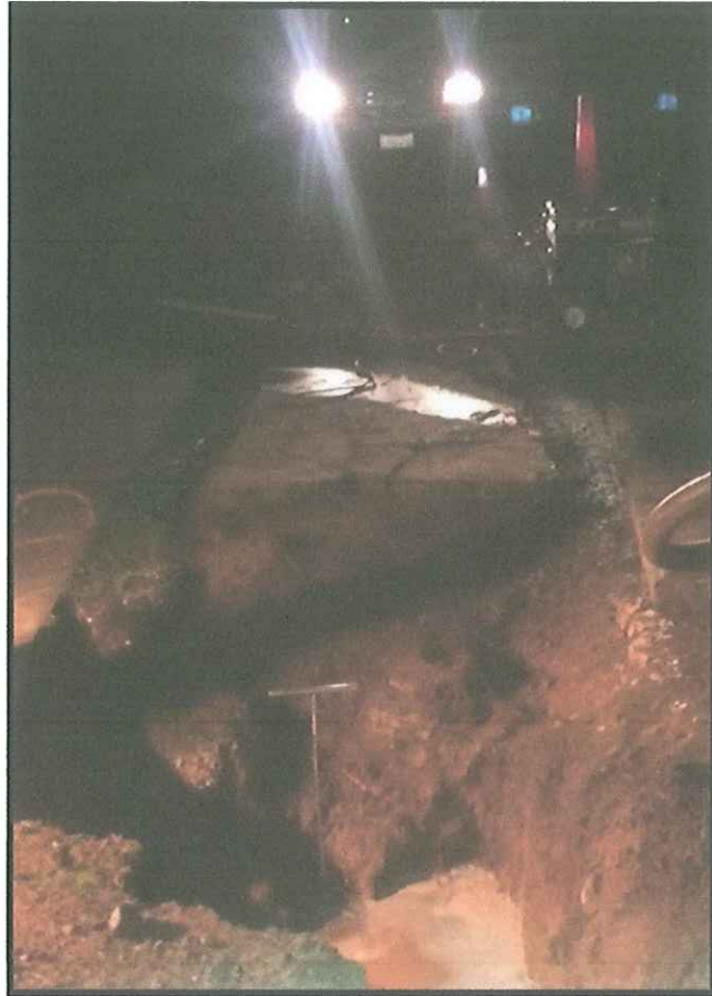
Emergency response to mainline break after hours.
