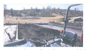
Cut open the geotubes and incorporated sludge into sludge bed maintenance.
