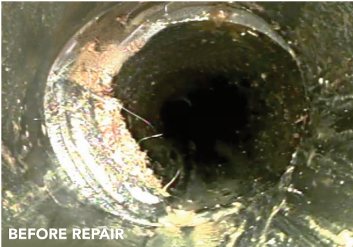
Sewer lateral (between main and house)
